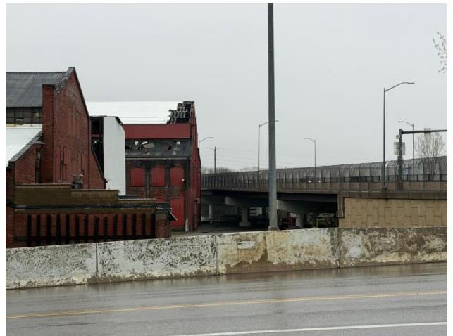
See visible damage and underpass of Erie Mill and Press Company Inc. by the highway.
