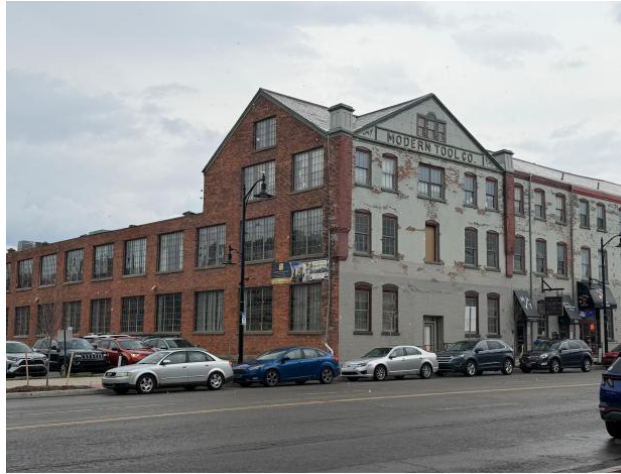
Modern Tool Co. is a repurposed factory made into apartment units.
